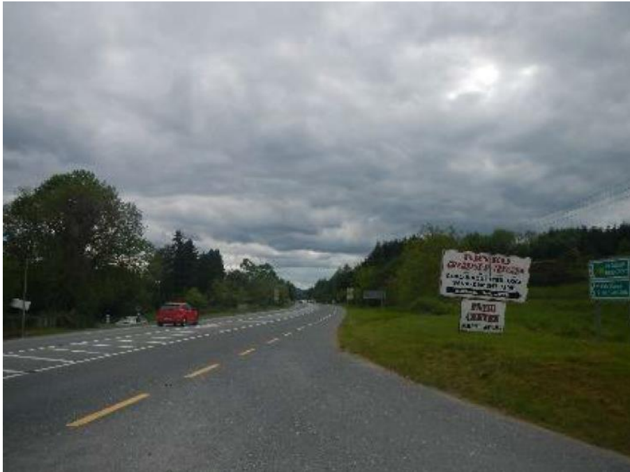
Figure 12.3 – N81 Looking South from Quarry Access
